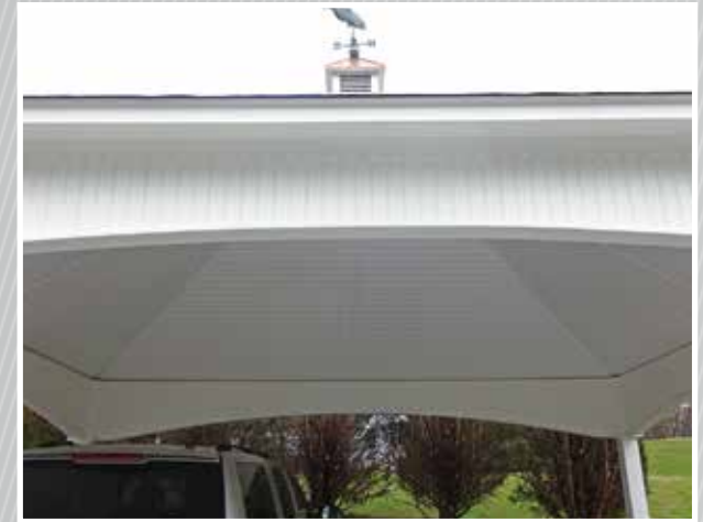
Dental Moulding and Bead Board Detail Header with Interior Vinyl Ceiling
