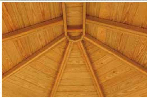
Interior ceiling with exposed rafters and tongue and groove underlayment.
