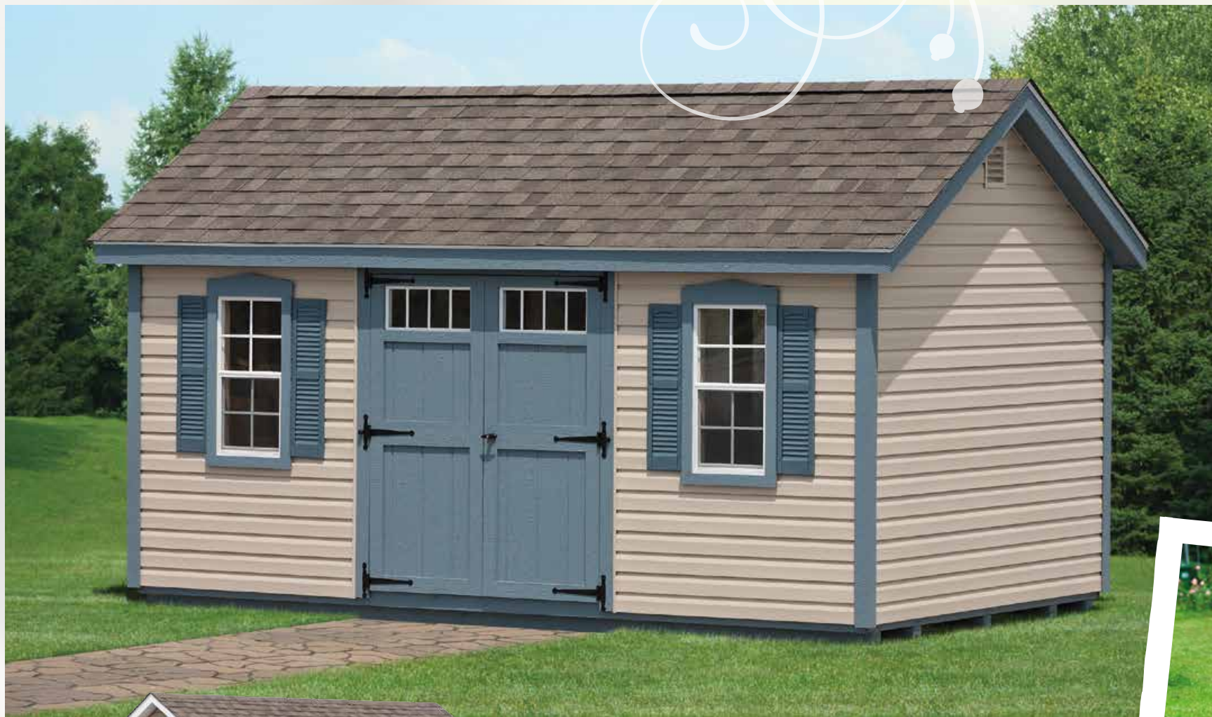
Wicker vinyl siding with weatherwood shingles
